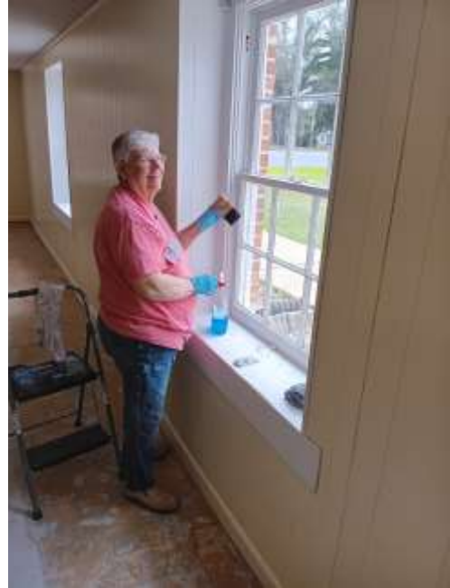
Painting the Window Frame
